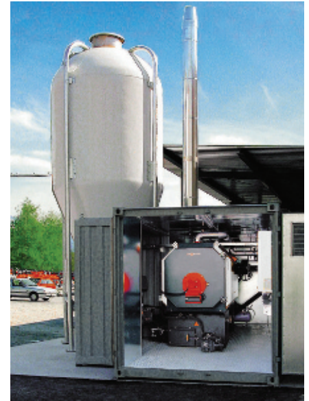
Portable boiler enclosure (pellet silo field supplied)
