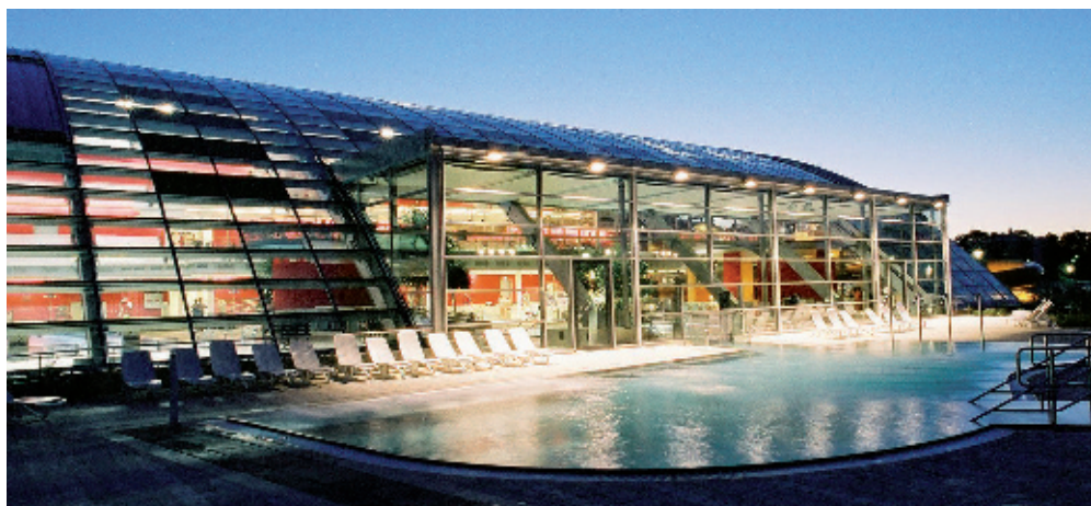
One of Germany's largest facilities powered by biomass heating technology. Recreational Pool and Spa. Kempten, Germany.
